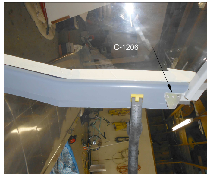
FIGURE 1: TRIMMING AFT END OF MOLDING
